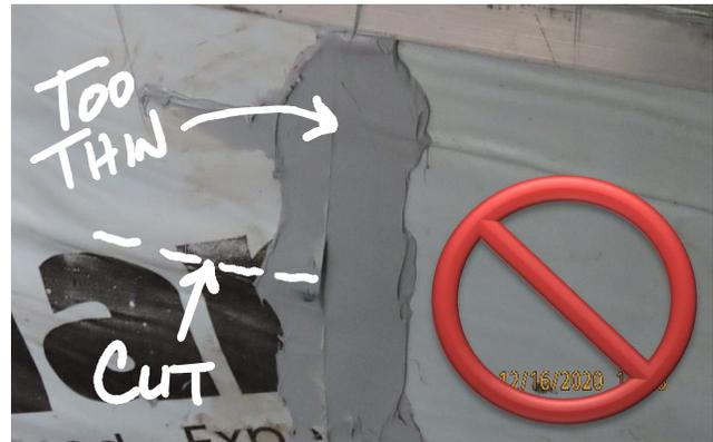
**Never just install sealant over a fish mouth...always slice the joint and properly roll and seal.**
